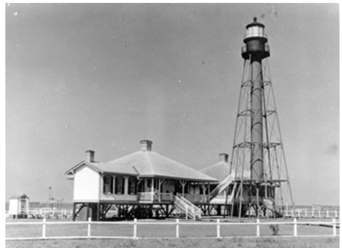
This lighthouse, built in 1896 at Velasco, helped guide ships to safety near the old mouth of the Brazos River. The Brazos Light was scrapped in 1967 after the property on which it sat was bought by Dow Chemical.
